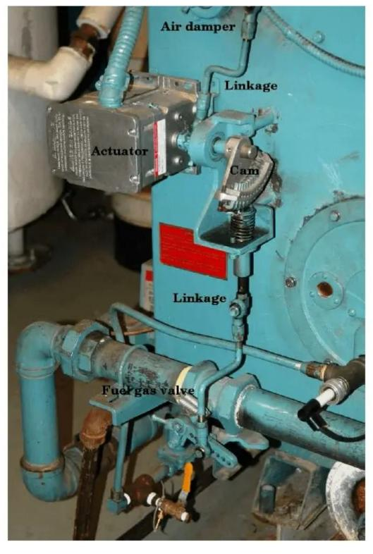
As you can see in this photo, the fuel gas valve is actuated by means of a cam, allowing precise "tuning" of the valve characteristics for consistent fuel/air ratio across a wide range of firing rates. Making ratio adjustments in such a linkage system is obviously a task for a skilled mechanic or technician.
